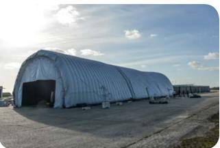
This is a unique solution for testing ADAS sensors in the dark. Exclusively available from Moshon Data, the sectional Inflatable Tunnel can be configured in various options.
